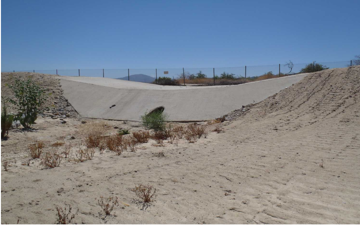
Basin inlet at the southeast corner of the basin.
