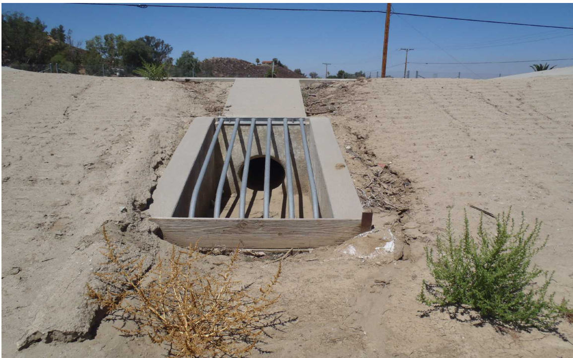
Basin outlet to Lake street at the northwest corner of the basin.
